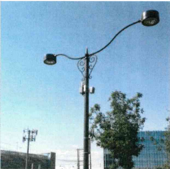
Light Pole Sound System for Town Audio
